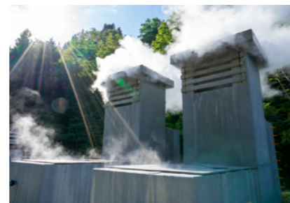
Fuming well in Tokamachi Geothermal Site
