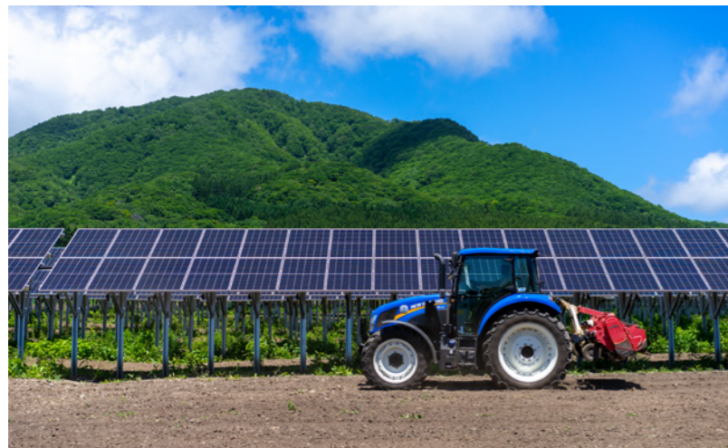
Oshamanbe Solar Powerplant
